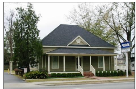
The Mill Foreman's house, now a professional office, is a frame vernacular building with Folk Victorian stylistic elements.
