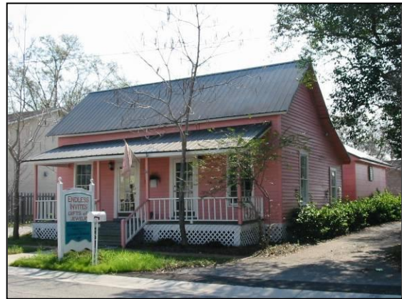
This retail shop (former mill worker's house) shows compatibility with several guidelines: façade materials, roof form, landscaping, and paving.
